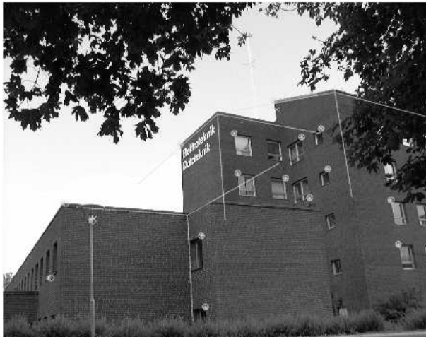
Figure 5: The three images used with three quivers. The reprojected points using the solution obtained from the quivers is also shown with original points as '*' and reprojected points as 'o'.
